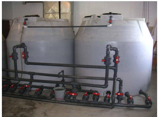
83" Biological Activated Carbon Filters
